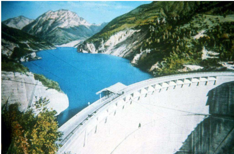
Figure 2a: The Vajont dam during impounding of the reservoir. In the middle distance, in the centre of the picture, is Mount Toc with the unstable slope visible as a white scar on the mountain side above the waterline.
