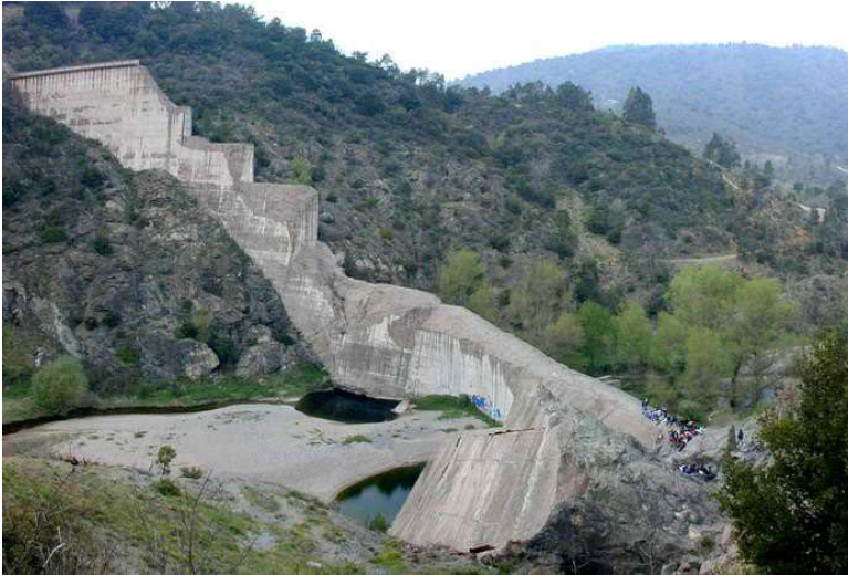
Figure 1: Remains of the Malpasset Dam as seen today. Photograph by Mark Diederichs, 2003.
