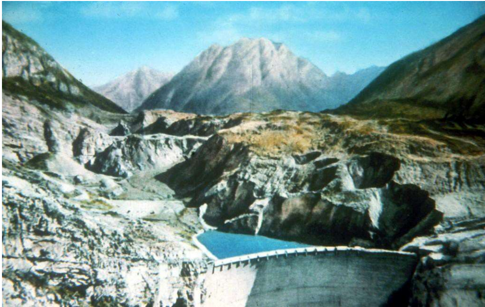
Figure 2b: During the filling of the Vajont reservoir the toe of the slope on Mount Toc was submerged and this precipitated a slide. The mound of debris from the slide is visible in the central part of the photograph. The very rapid descent of the slide material displaced the water in the reservoir causing a 100 m high wave to overtop the dam wall. The dam itself, visible in the foreground, was largely undamaged.
