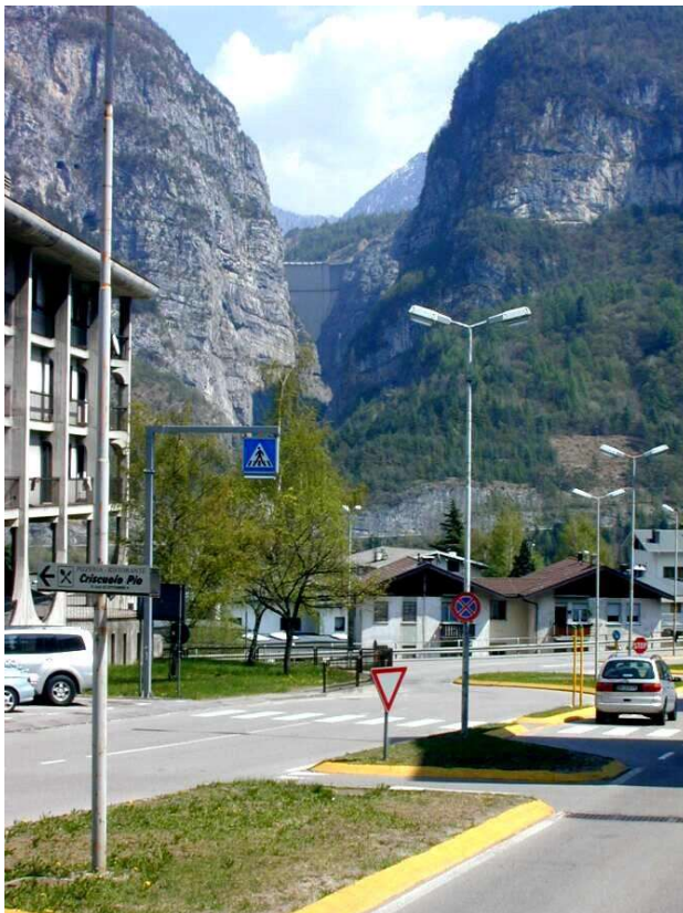
Figure 2e: The remains of the Vajont dam perched above the present town of Longarone. Photograph by Mark Diederichs, 2003.
