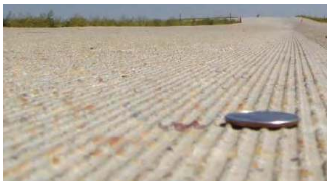
Figure 5.11 Diamond-ground texture (Rasmussen et al. 2008)
