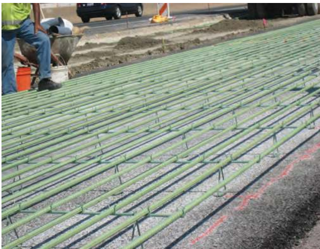
Figure 4.10 Reinforcing for CRCP (photo courtesy of Mike Ayers, American Concrete Pavement Association)
