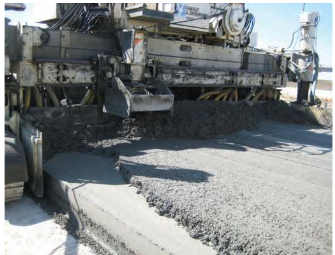
Figure 3.2 Two-lift pavement being constructed in Kansas
