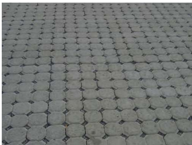
Figure 3.5 Permeable interlocking concrete paver blocks make an aesthetically pleasing, well-drained pavement for low-volume streets and parking lots (photo courtesy of Interlocking Concrete Pavement Institute)
