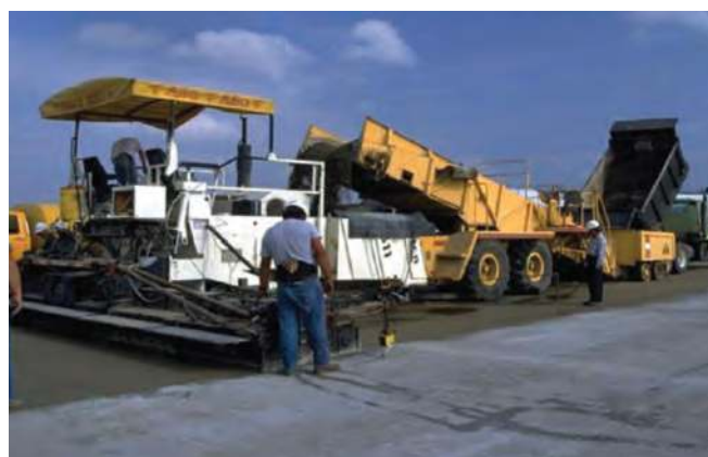
Figure 5.14 RCC placement (Harrington et al. 2010)
