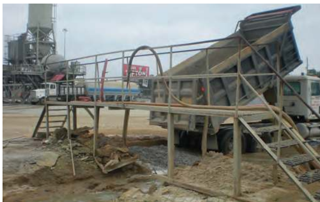
Figure 5.8 Washout pit used to clean concrete trucks (photo courtesy of Gary Fick, Trinity Construction Management, Inc.)
