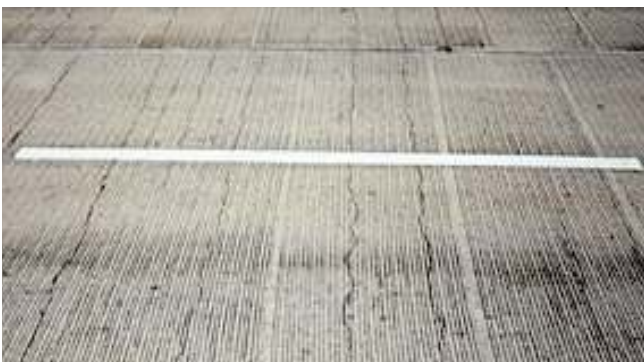
Fig. 6-17. Shrinkage cracks, such as shown on this bridge deck, can be reduced with the use of good concreting practices and shrinkage reducing admixtures. (69883)
