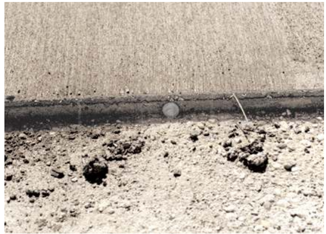
Fig. 6-10. Plasticized, flowing concrete is easily placed in thin sections such as this bonded overlay that is not much thicker than 1\frac{1}{2} diameters of a quarter. (69874)
