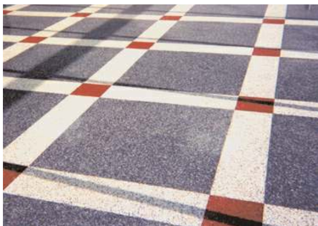
Fig. 6-19. Red and blue pigments were used to color this terrazzo floor. (69873)
