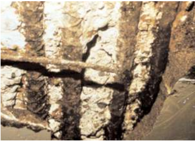
Fig. 6-16. The damage to this concrete parking structure resulted from chloride-induced corrosion of steel reinforcement. (50051)
