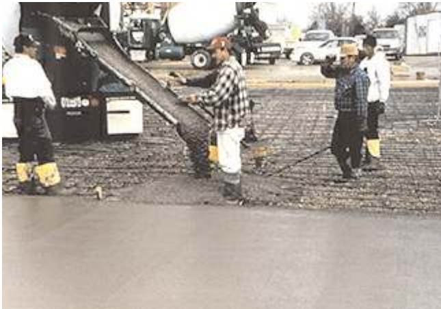
Fig. 6-10. Plasticized, flowing concrete is easily placed in thin sections such as this bonded overlay that is not much thicker than 1\frac{1}{2} diameters of a quarter. (69874)
