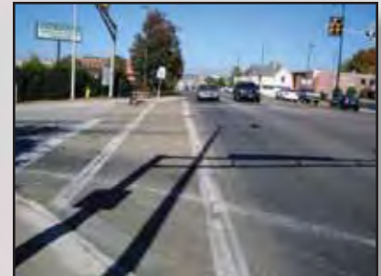
Unnecessarily large curb radii result in longer pedestrian cross times, higher vehicle speeds, and reduced visibility.
