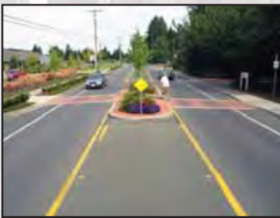
A 'Z' configuration causes pedestrians to face oncoming traffic at mid-block crossing locations.
