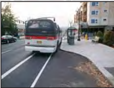
Bus bulb-outs are preferred over turn-outs because they provide higher visibility and do not require transit vehicles to exit and re-enter the traffic stream.
