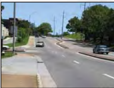
Raised medians provide a safer refuge (compared to a flush median) for pedestrians and break one complex crossing into two simpler ones.
