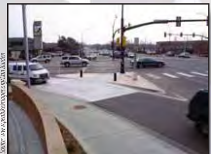
Channelizing islands improve pedestrian visibility and shorten crossing distances, but must be carefully designed so that they do not result in faster motor vehicle turn movements.
