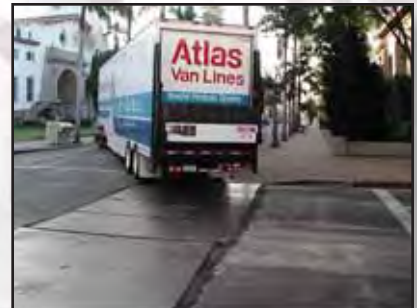
It's OK to have smaller curb radii where larger vehicles do not turn often.
