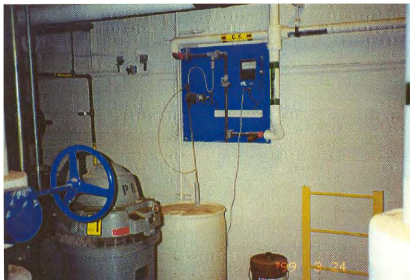
Figure 7-4. Automatic Neat Chemical Feed
