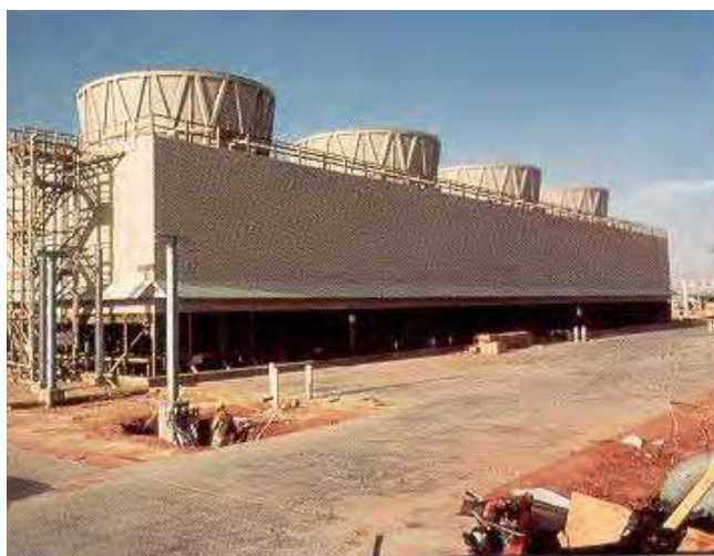
Figure 4-9. Counter-Flow Cooling Tower
