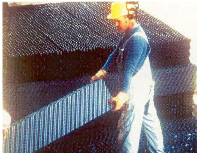
Figure 4-11. High-Efficiency Cooling Tower Film Fill
