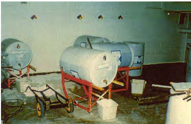
Figure 7-2. Manual Chemical Feed System
