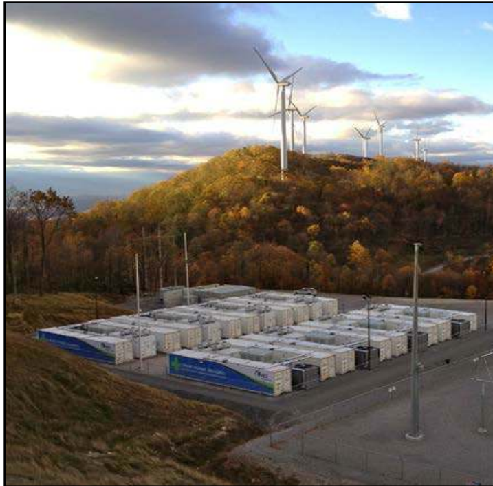
Figure 97. AES Storage LLC's Laurel Mountain Energy Storage (Supplies 32 MW of regulation in PJM using Li-ion batteries supplied by A123 Systems)
