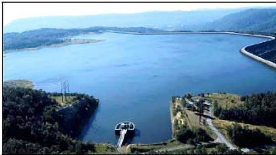
Figure 21. Man-made Upper Reservoir of TVA's Raccoon Mountain Pumped Hydro Plant (Operational in 1979, the facility can generate 1620 MW for up to 22 hours.)
