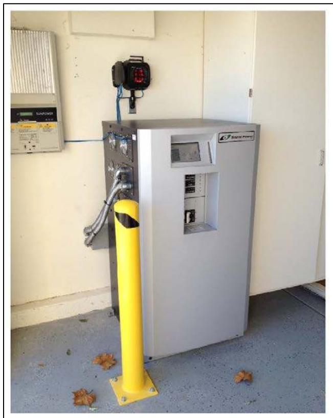
Figure 100. Residential Energy Storage and Energy Management Systems
