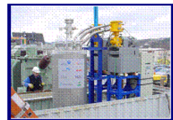
CURL 10 Fault Current Limiter
