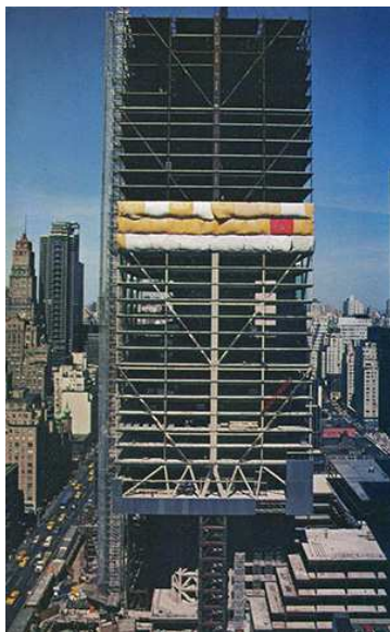
Figure 4: Citicorp tower under construction
