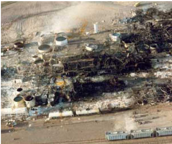
Remnants of the PEPCON facility
