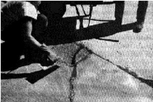
Figure 4. Finishing a patch containing an active crack.
