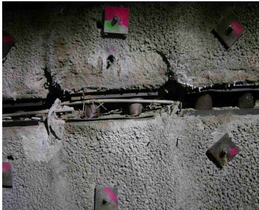
Figure 8-4 Yielding Support Crushed to 20 cm (One-half) (ILF, 2008)
