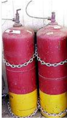
Figure 4. Properly stored cylinders
