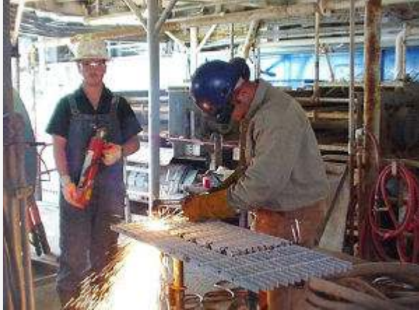
Figure 1. Hot work - welding
