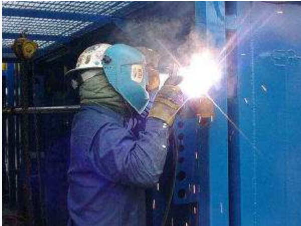
Figure 3. Welding - hot work
