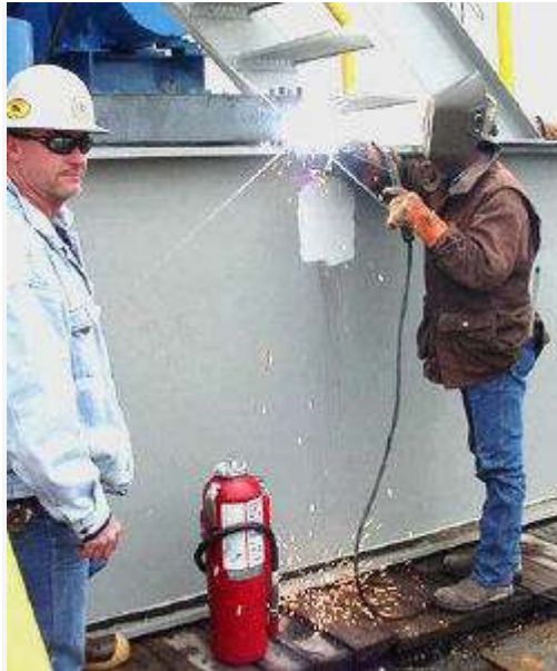
Figure 2. Welding with fire control
