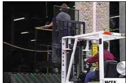
Figure 6. Specialized platform for lifting coworker.
