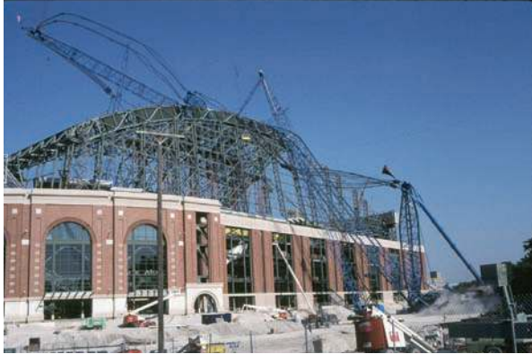
Figure 2. Heavy-lift crane after tip-over at stadium project. (Photo courtesy of John Thraen)
