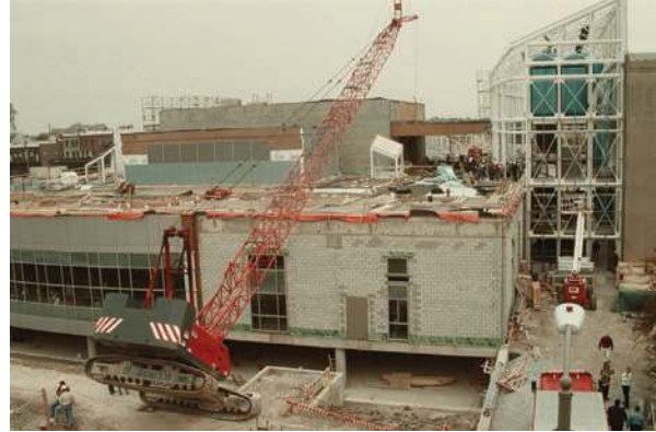
Figure 3. Crane tip-over at library expansion project. (Photo courtesy of The Blade/Toledo Ohio)
