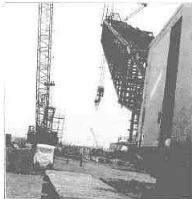
CRAWLER CRANE PREPARED FOR INSPECTION
