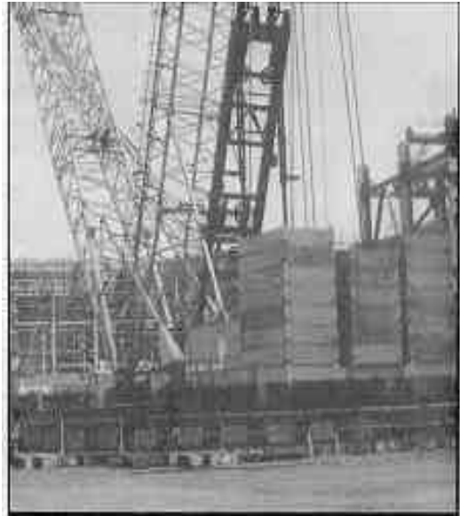
MODERN RINGER CRANE 500 TON CAPACITY
