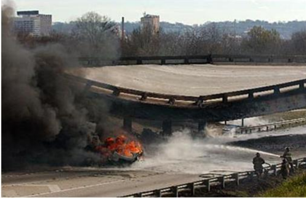
Figure 6 Fuel truck crash causes severe fire under the I-65 South over I-65 North overpass in Birmingham, Alabama, January 2002.
