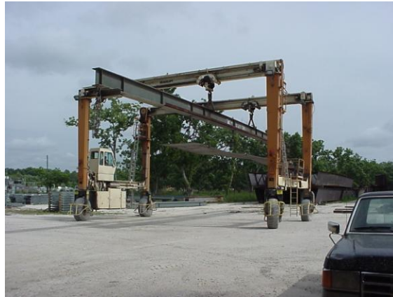
Figure 10 Photo showing overhead gantry type cranes handling material
