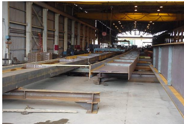
Figure 12 Photo taken in a fabrication shop showing the fitting of transverse stiffeners
