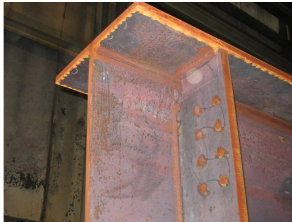
Figure 16 Photo showing a girder before blast cleaning
