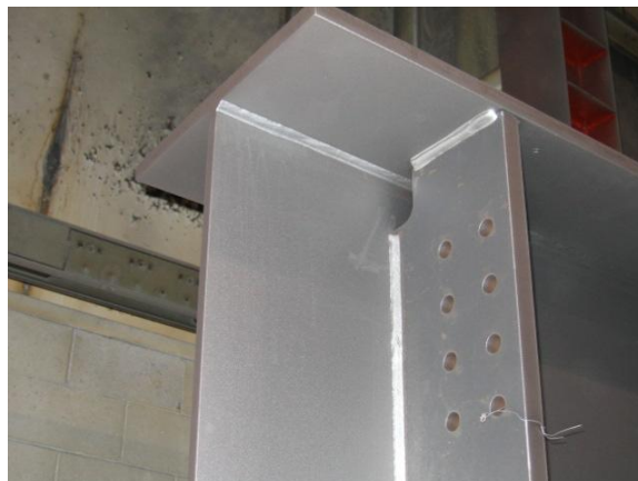
Figure 17 Photo showing a girder after blast cleaning
