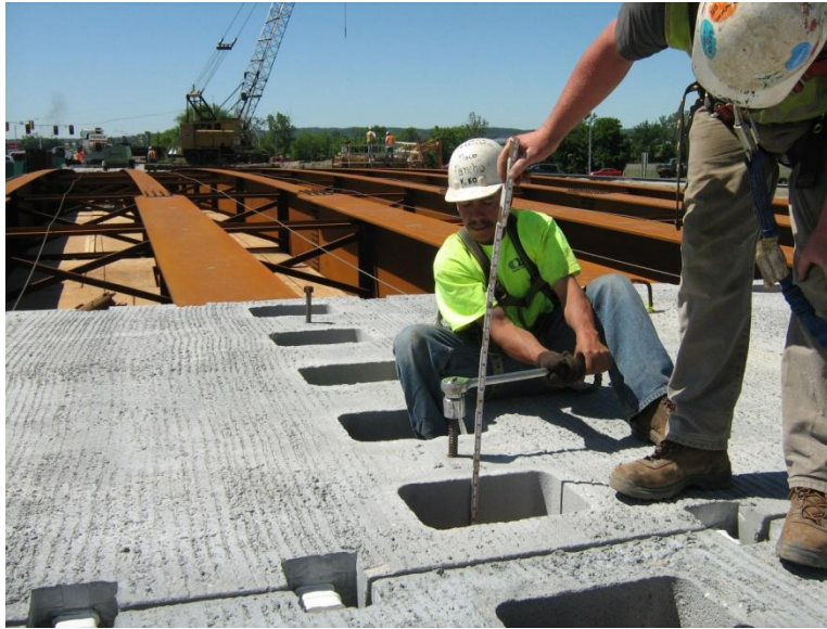
Figure 2 Construction workers adjusting the elevation of the full depth precast concrete deck panels by adjusting leveling bolts (courtesy Iowa DOT).
