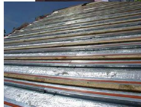
The battens not only provided a casing for the solar product, they also solved another problem: the stability of the roof frame and the uneven deck. The battens leveled the roof and provided structural integrity and shear strength.
