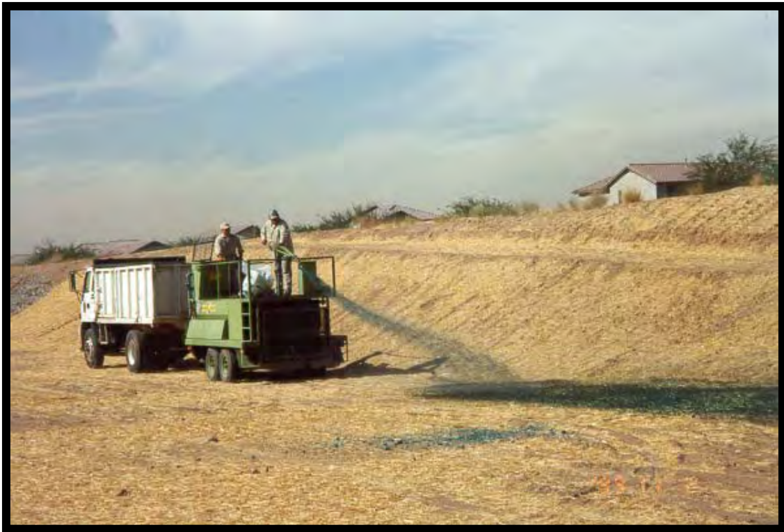
Figure 8. Hydro-seeding operations on a floodway dam in Maricopa County, Arizona (Renckly & Drake, 1999).
