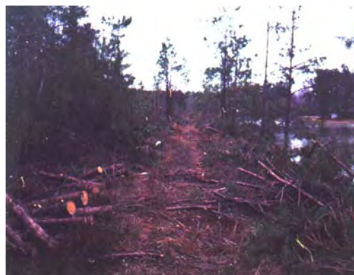
Figure 6. Trees cut prior to removing stumps and roots from dam.
