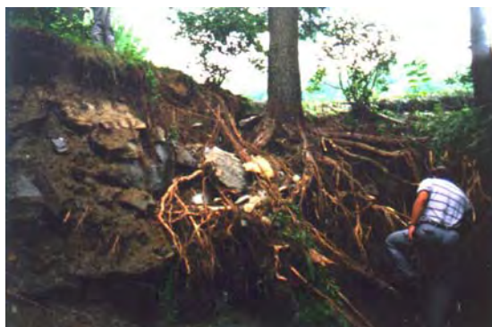
Figure 6. Tree root induced scouring on crest and downstream face of Coffey dam in Kansas.
