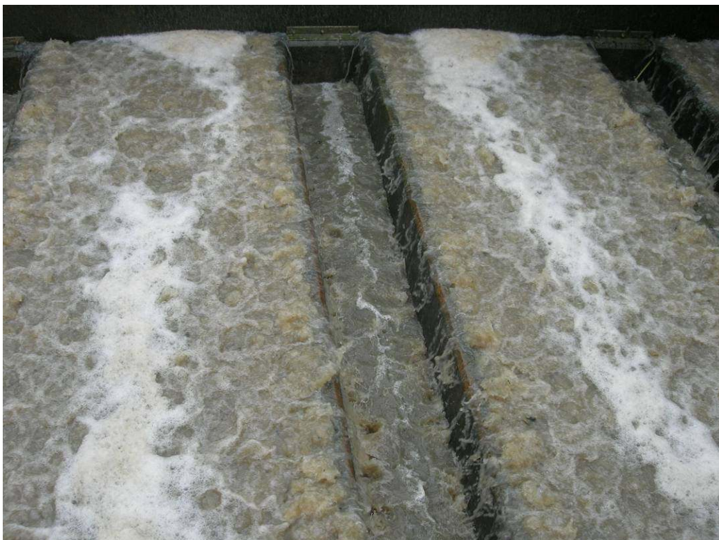
Bed filter undergoing backwash at Alexandria AWWTP
