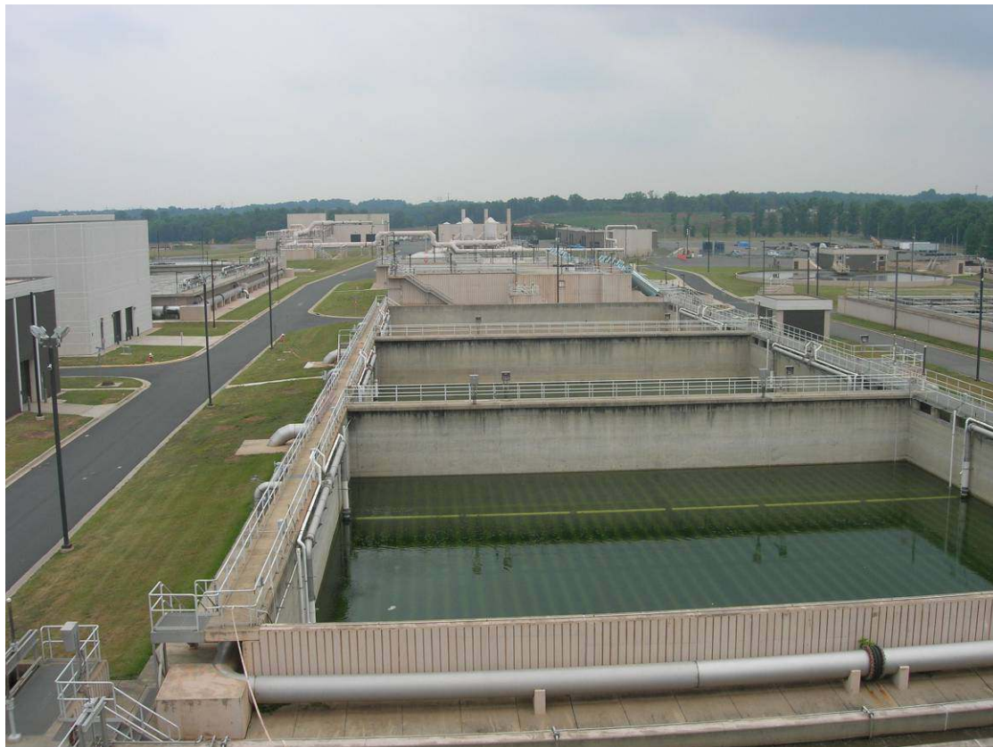
UOSA Water Reclamation Facility (WRF) – in the forefront are fine bubble diffuse aeration basins constructed during the plant expansion to 27 mgd which are off-line in this picture.
