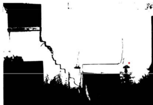
b. Diagonal and vertical cracks
