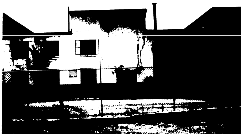
a. Vertical cracks
