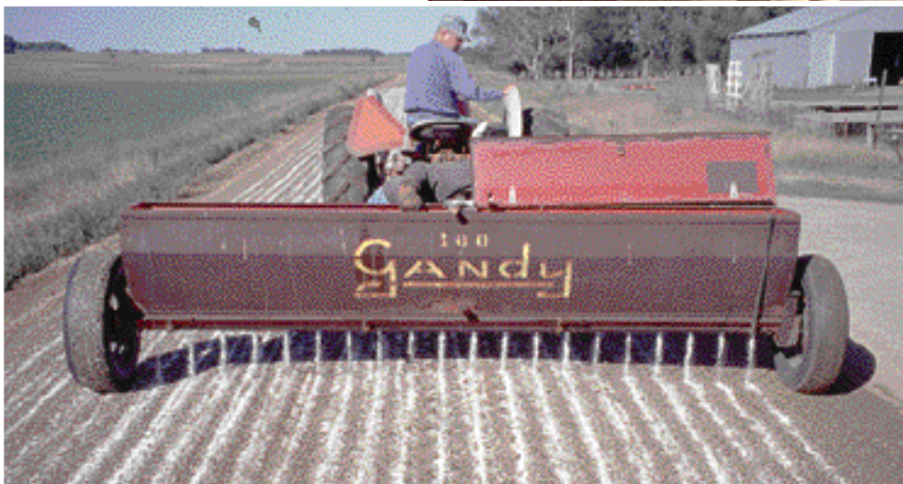
This photo shows part of the spray bar with spraying nozzles.
