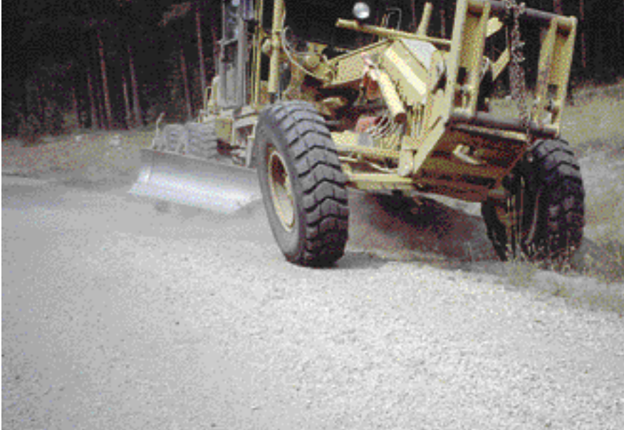
An example of work with a grader to reshape a ditch on a mountain road.
