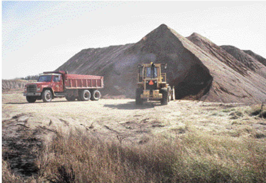
A good example of loader operation — working uniformly across the end of the stockpile. Note also a very level stockpile site and a well maintained loading area on which the loader and trucks work. This demonstrates pride in doing a good job of handling material.
