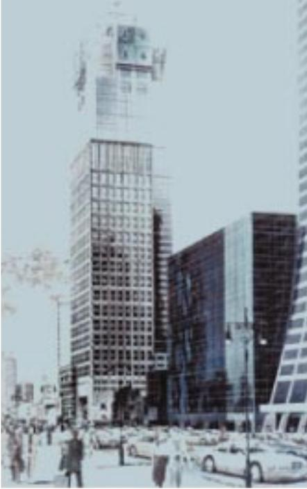
*4 Times Square in New York City is one of the first office buildings in the U.S. to be powered by a 200 kW phosphoric acid fuel cell system*
