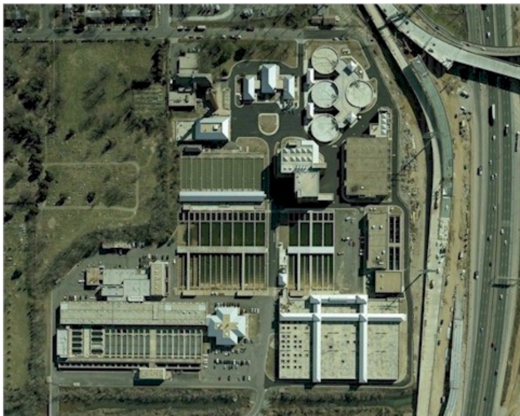
Aerial View on ASA Advanced Wastewater Treatment Facility (from ASA staff)
