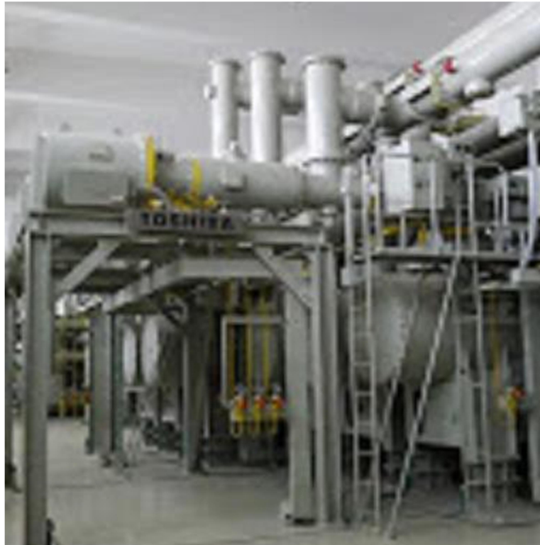
Figure 6. SF6 gas to air bushings
