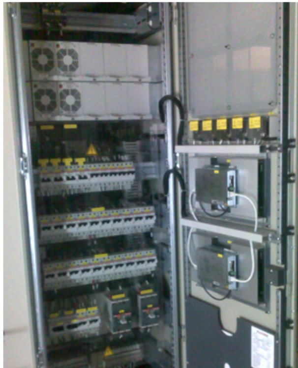
Figure 21. Busbar protection relay using the latest numerical technology
