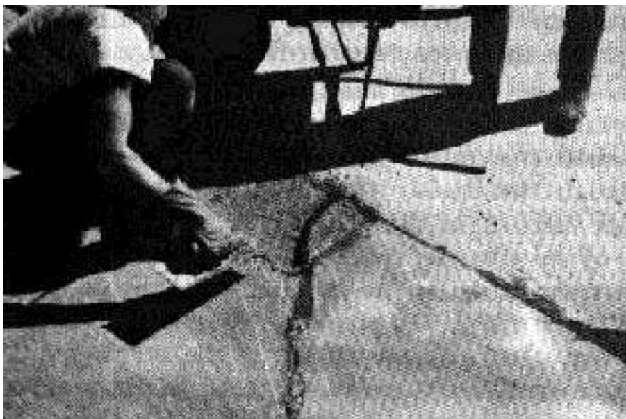
Figure 4. Finishing a patch containing an active crack.
