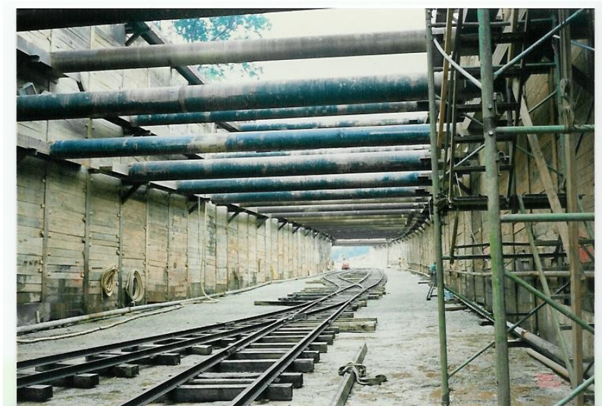
Figure 5-5 Braced Soldier Pile and Lagging Wall
