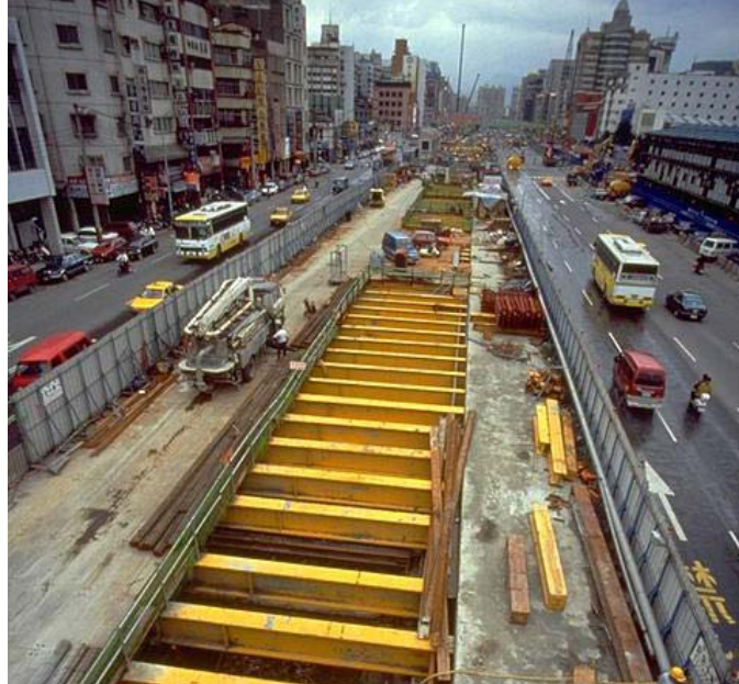
Figure 5-7 Braced Slurry Walls
