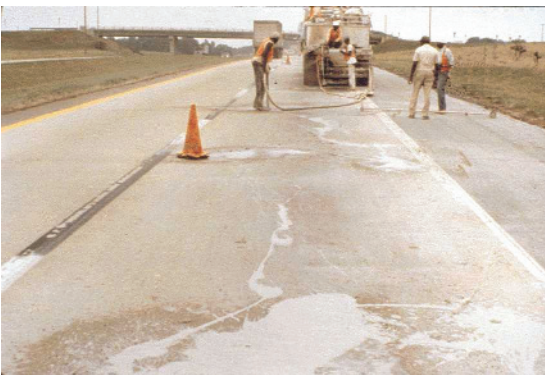
Figure 9-1. Fly ash grouts for pavement subsealing
