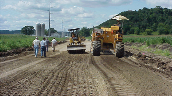
Figure 7-1. Mixing and shaping of fly ash stabilized soil.
