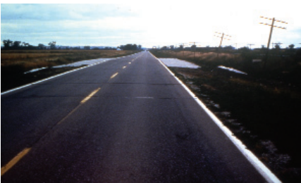
Figure 5-5. Bridge replaced by culverts and flowable fill.
