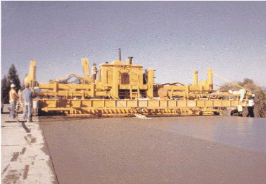
Figure 3-1. Fly ash improves workability for pavement concrete.
