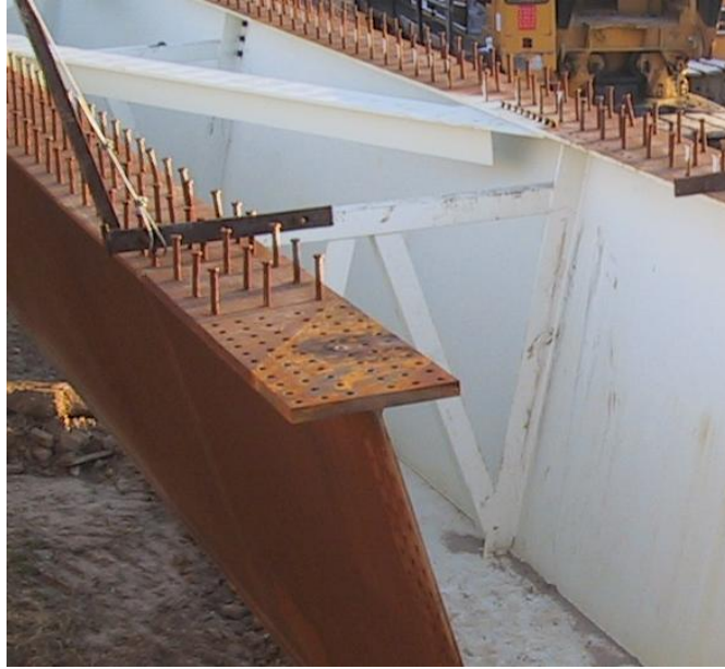
Figure 59 Strut offset below diagonal
