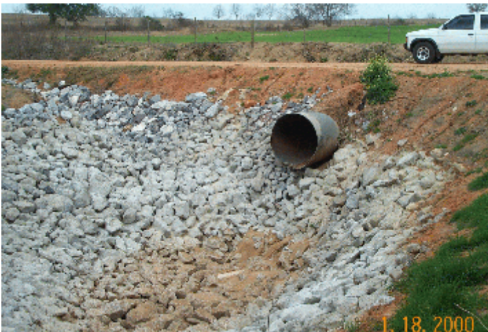
Exhibit 3.1b - Culverts for Crossing Natural Drains
