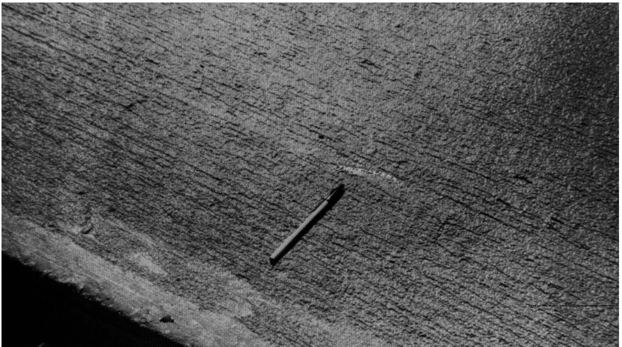
FIGURE 2-4. HEAVY BURLAP DRAG FINISH
