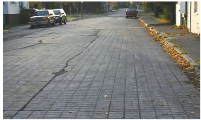
Figure 9.4 Blome Granitoid concrete pavement constructed in 1906 in Calumet, Michigan; the brick pattern was stamped into the surface to keep horses from slipping (photo courtesy of Tom Van Dam, CTLGroup)
