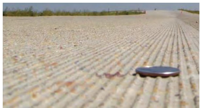
Figure 5.11 Diamond-ground texture (Rasmussen et al. 2008)
