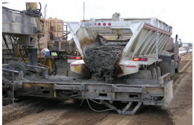
Figure 5.7 Tractor trailer concrete hauling unit (photo courtesy of Gary Fick, Trinity Construction Management, Inc.)
