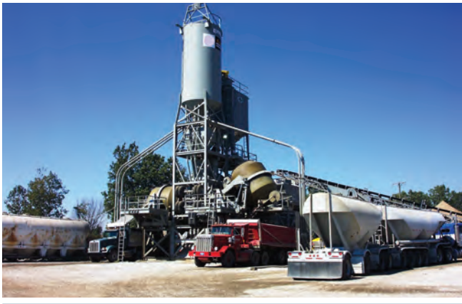
Figure 5.4 Central mix concrete plant (photo courtesy of Jim Grove, FHWA)
