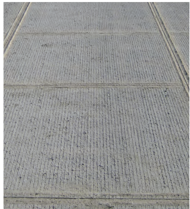
Figure 7.11 Unbonded overlay
