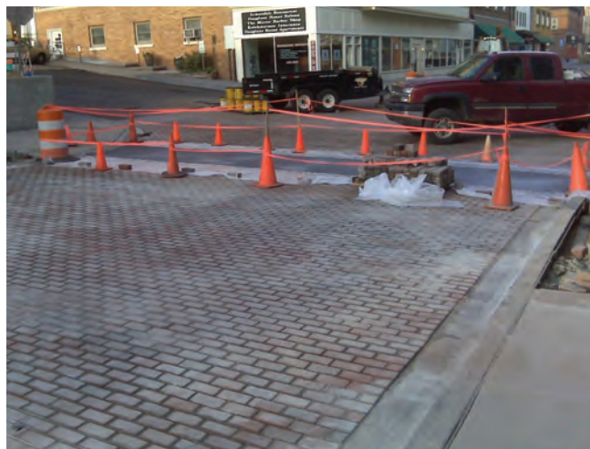
Figure 3.6 Vehicular interlocking concrete pavers being placed in a historic downtown area (note the use of colored concrete to provide a visual offset for the crosswalk) (photo courtesy of Tom Van Dam, CTLGroup)
