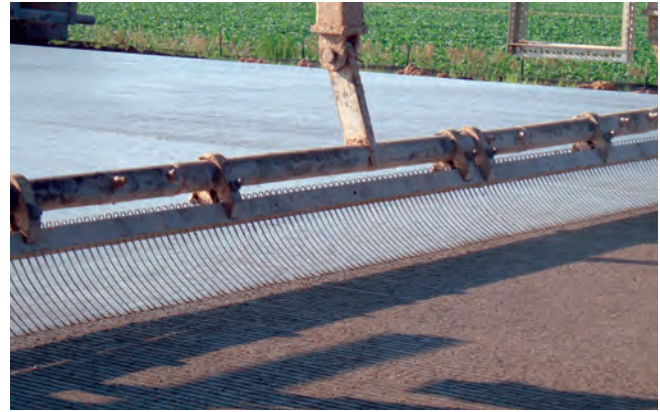
Figure 5.9 Longitudinal tining (photo courtesy of Gary Fick, Trinity Construction Management, Inc.)
