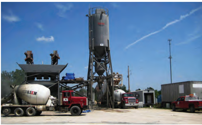
Figure 5.5 Ready mix concrete plant (photo courtesy of Jim Grove, FHWA)
