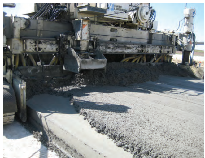
Figure 3.2 Two-lift pavement being constructed in Kansas
