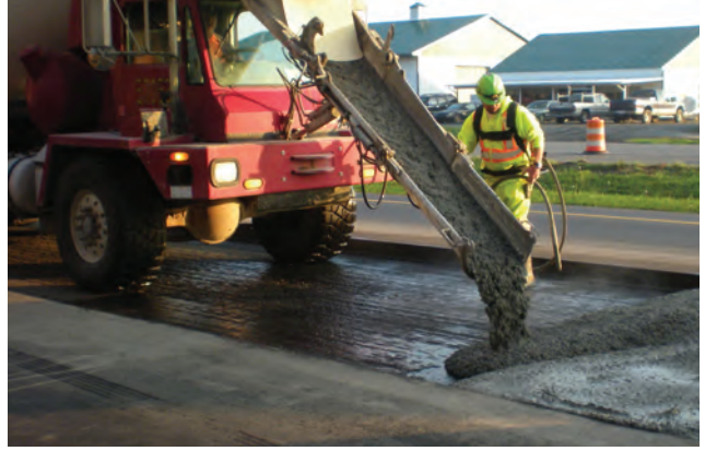
Figure 5.6 Transit mix concrete truck (photo courtesy of Gary Fick, Trinity Construction Management, Inc.)
