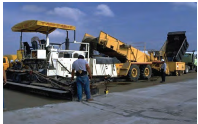
Figure 5.14 RCC placement (Harrington et al. 2010)
