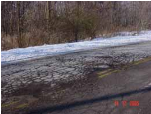
Figure 8: Roughness due to severe cracking.
