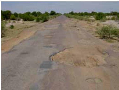
Figure 8: Roughness due to severe cracking.
