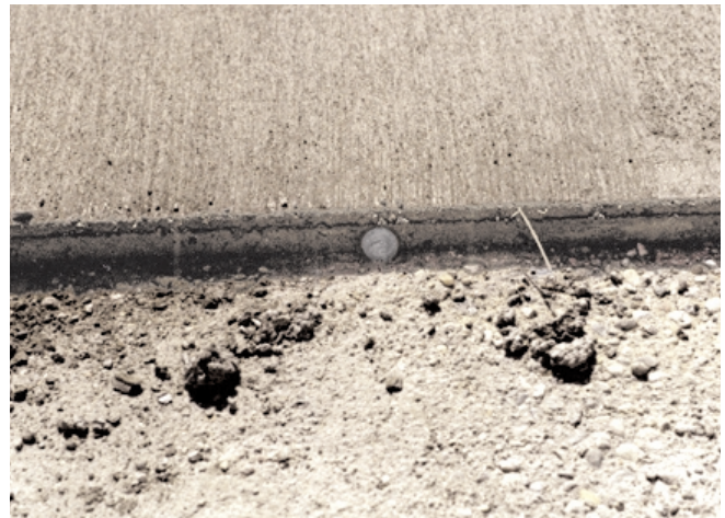
Fig. 6-10. Plasticized, flowing concrete is easily placed in thin sections such as this bonded overlay that is not much thicker than 1½ diameters of a quarter. (69874)
