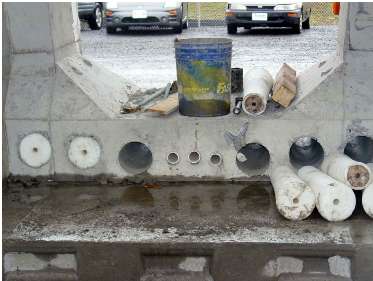
Figure 2.12 - Reusable Diabolo Inserts at Deviation Segment
