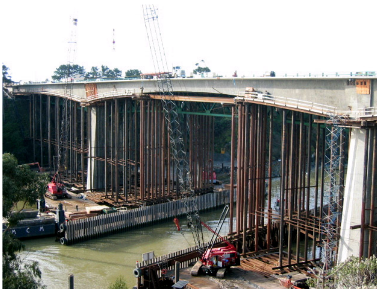
Figure 1.6 - Cast-In-Place Post-Tensioned Construction in California
