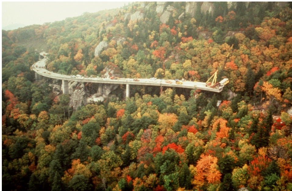
Figure 1.23 - Progressive Construction of the Linn Cove Viaduct
