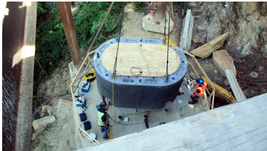
Figure 1.32 - Precast Hollow Segmental Piers, Foothills Bridge No. 2
