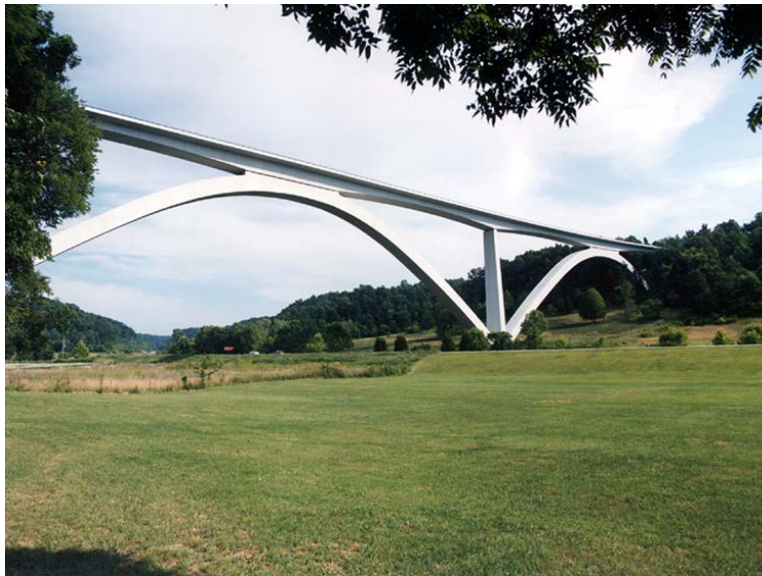
Figure 1.34 - Natchez Trace Parkway Arches, Tennessee
