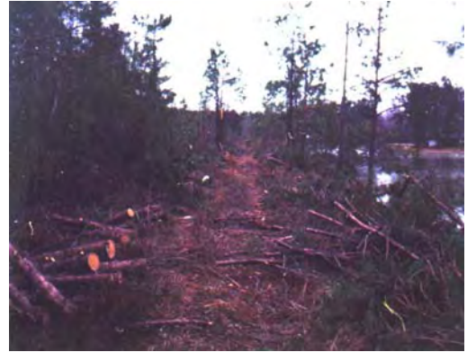
Figure 6. Trees cut prior to removing stumps and roots from dam.
