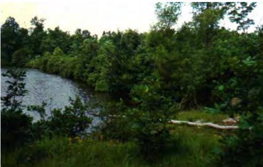
Figure 3. Example dam with inspection-hindering trees in Tennessee.
