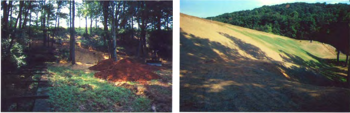
Figure 1. Restored Downstream Slope on Fishing Creek Dam, Maryland (1991-92)
