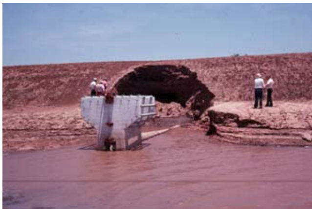
Figure 45-1 Failed embankments
