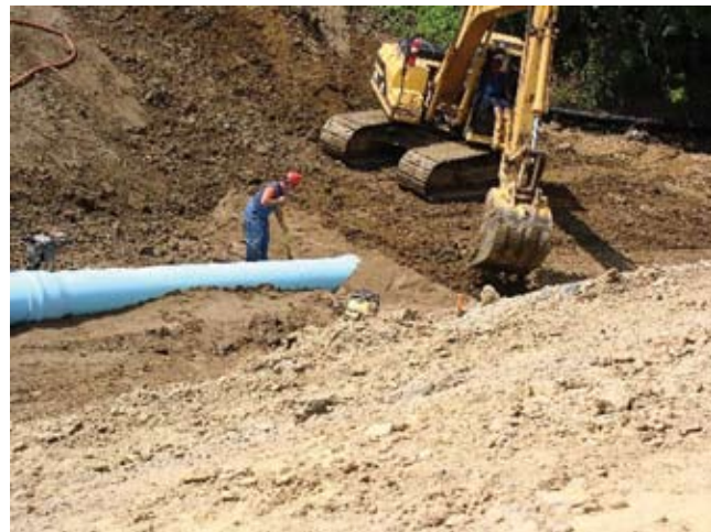
(f) Filter diaphragm being constructed above and to both sides of large diameter flexible pipe
