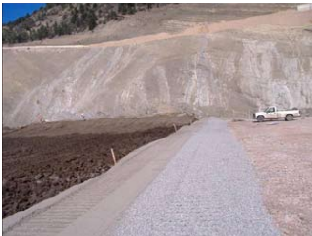
(g) Earthfill is compacted on both sides of the filter zones that have been laid. The process is then repeated as the embankment is raised.
