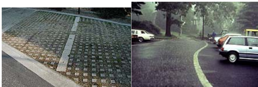
Fig. 20 (left): Belgium block pavers in parking bays and Fig. 21. (right): Permeable parking bays
