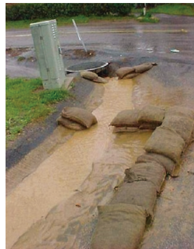
Figure 5. Make sure storm drain inlets are protected.
