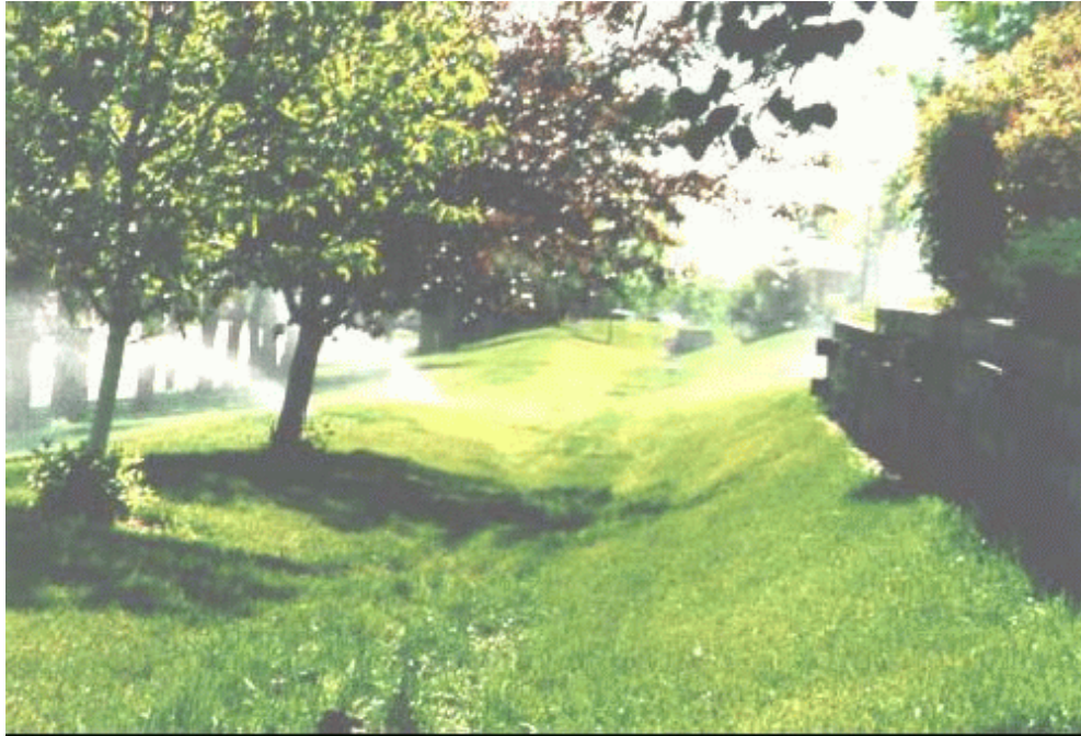
Figure 6-4 Typical Grass Swale (UDFCD, 1999)
