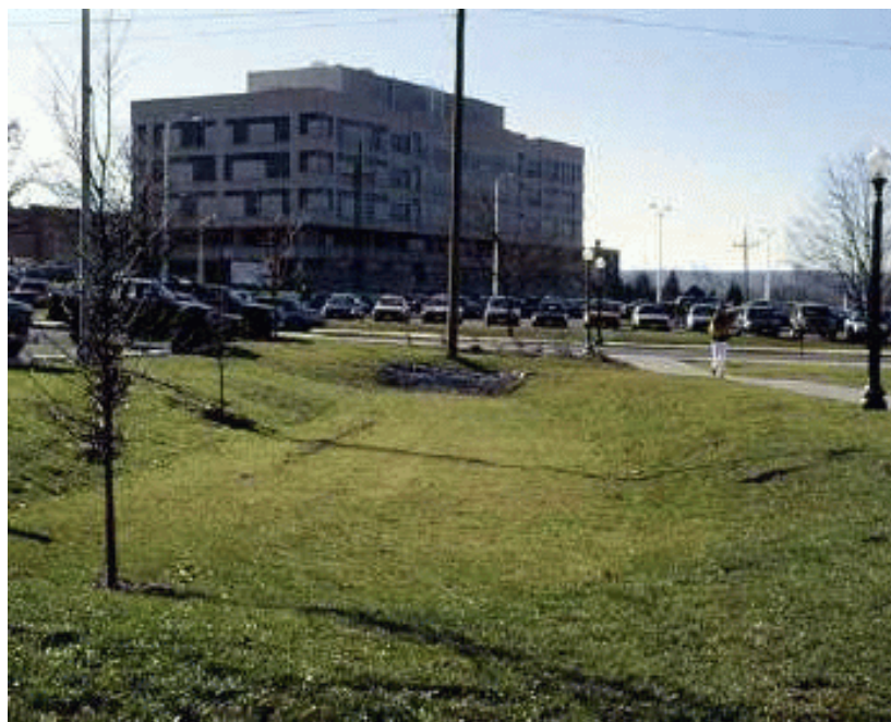
Figure 6-2 Grass Swale with Check Dam (VA DEC, 1999)
