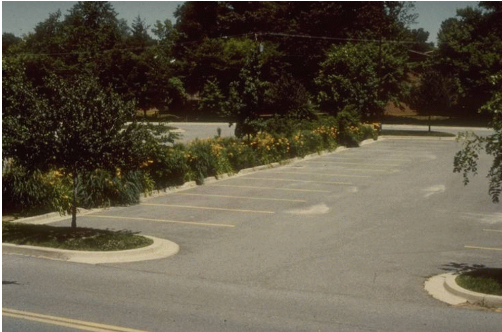
Figure 7-3 Bioretention Application on New Parking Lot
