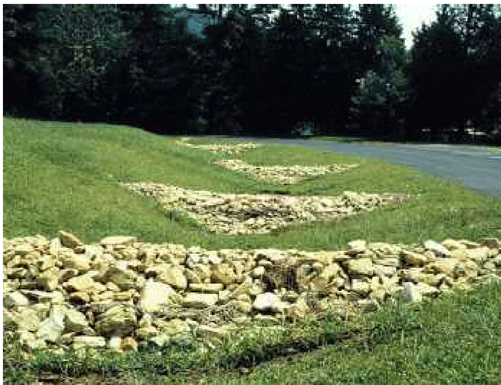
Figure 6-3 Grass Swale with Check Dams (VA DEC, 1999)
