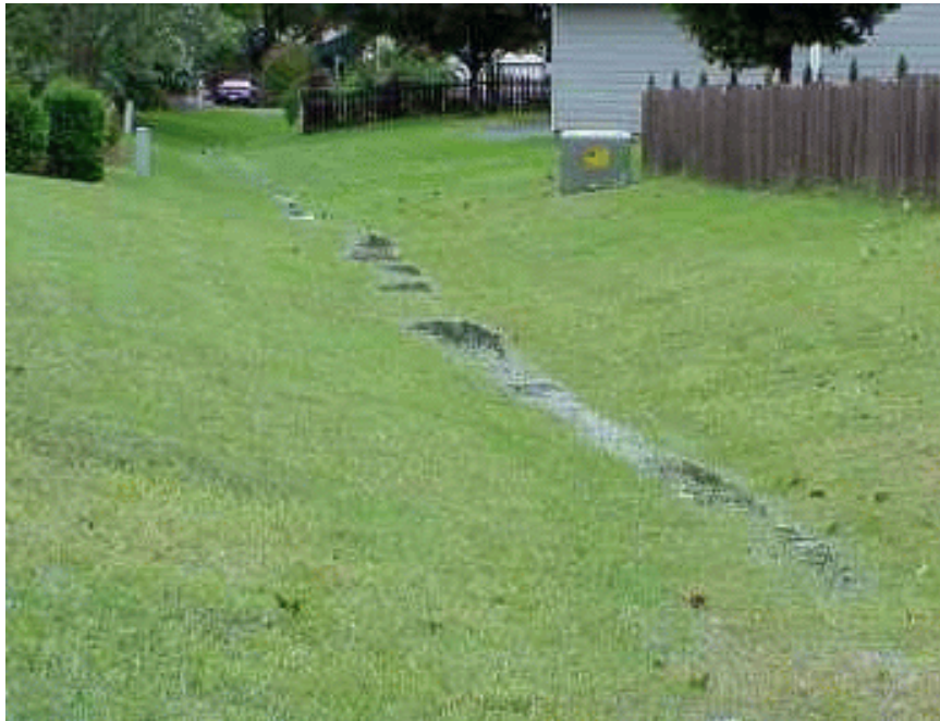
Figure 6-1 Grass Swale (VA DCR, 1999)
