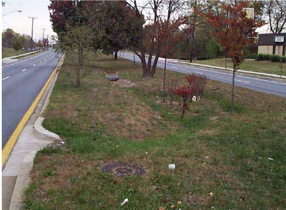
Figure 7-5 Bioretention Application in a Roadway Median
