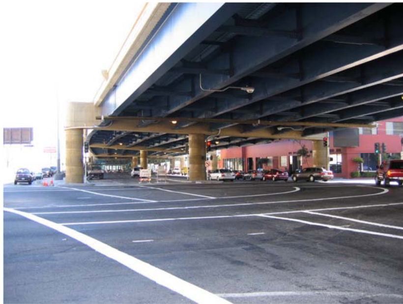
Figure 9.1-1 Central Viaduct in San Francisco
