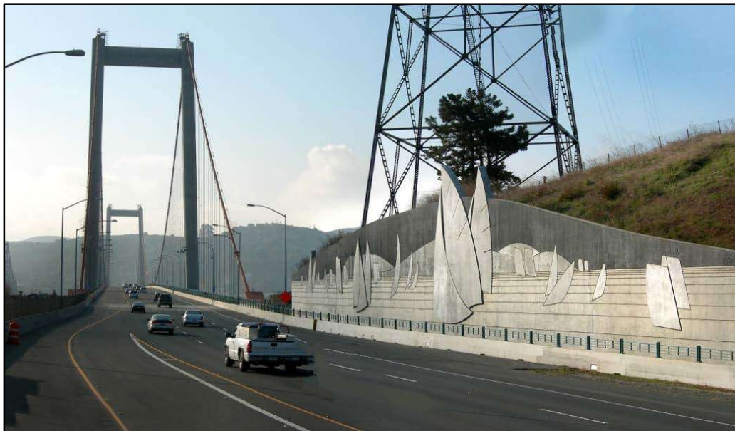
Aesthetic treatments on wall structures can reflect an image of the surrounding community and create visual interest for motorists.
