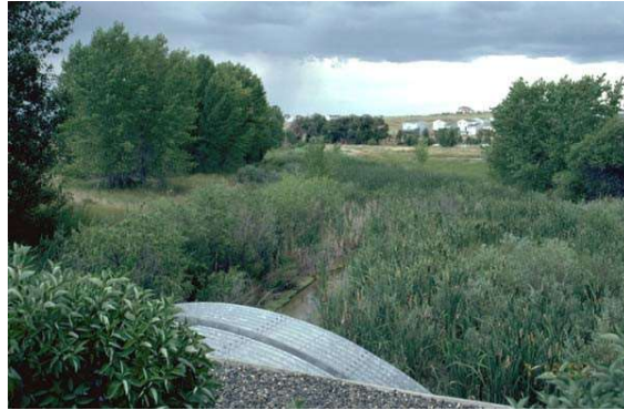
Photograph CU-2—Culverts can be designed to provide compatible upstream conditions for desirable wetland growth.
