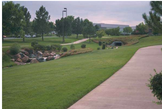
Photograph CU-3—Culverts can be integrated into the urban landscape without negative visual impact.
